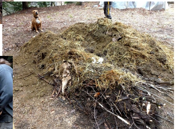
Finally the dirt that had been dug out for the hole was added on top and
